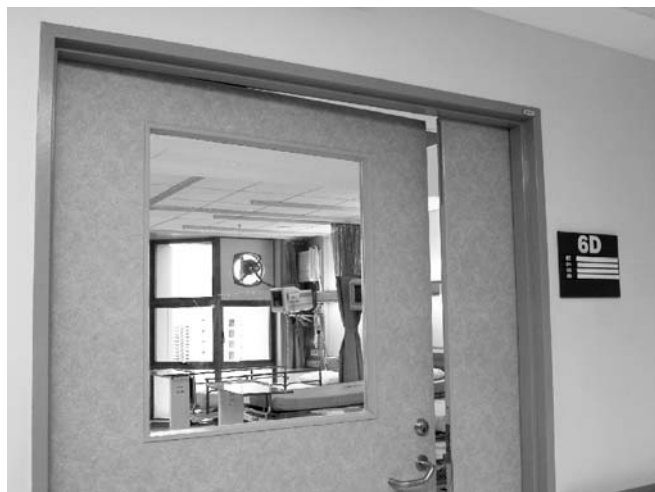
Fig. 1 An industrial fan mounted in a window can be used to create negative pressure. Mounting at floor level is preferable if this does not create a hazard. Door springs can be adjusted so that the door remains ajar when the exhaust fan within the room is operating normally. This provides a crude method for monitoring air changes
